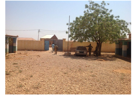
View of entrance gate (beyond). There is also a flag pole with a concrete cast base.
