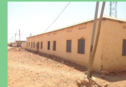
The existing building has windows opening outwards along the parcel boundary.
