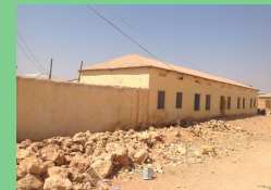
External view of the main structure and boundary wall.
