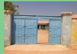
View of the entrance gate.
