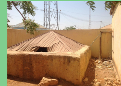
View of the existing water storage tank.
