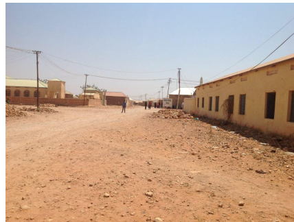
There are roads on three faces of the site.
