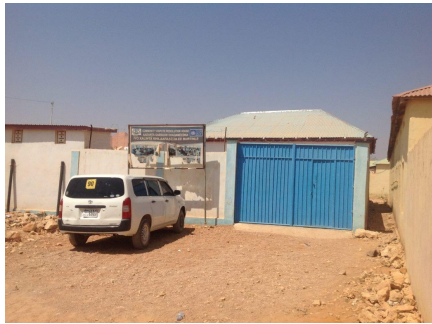
View of the closest neighbour; the site's boundary wall is on the right.
