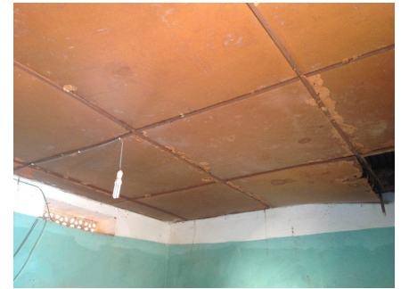
View of existing ceiling and electrical installation.
