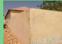
View of the existing 2m high boundary wall.
