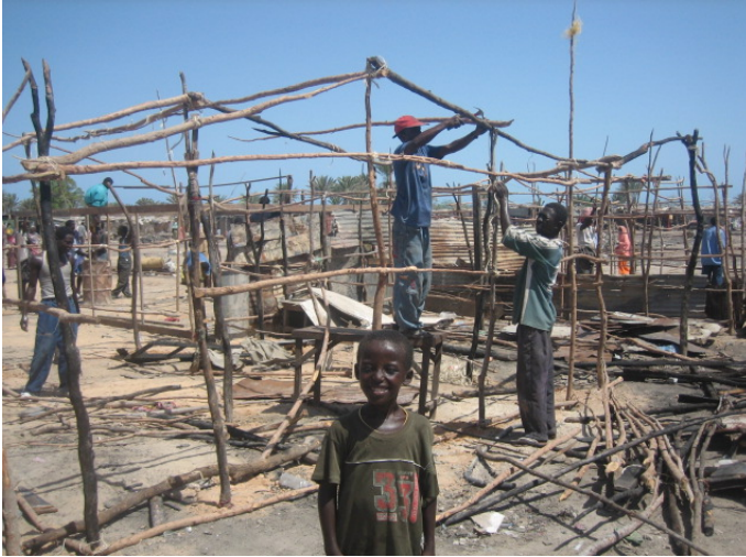
Inhabitants of 'Boqolka Bush' IDP settlement rebuilding their buuls . Source: Joana Cameira, UN-HABITAT.
